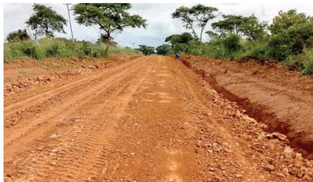
Znbs constructed community road in Balmoral area in Chilanga district.
