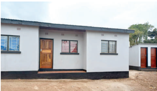
Sponsored the construction of a community house for a vulnerable family in collaboration with Habitat for Humanity in Mapepe, Chilanga district
